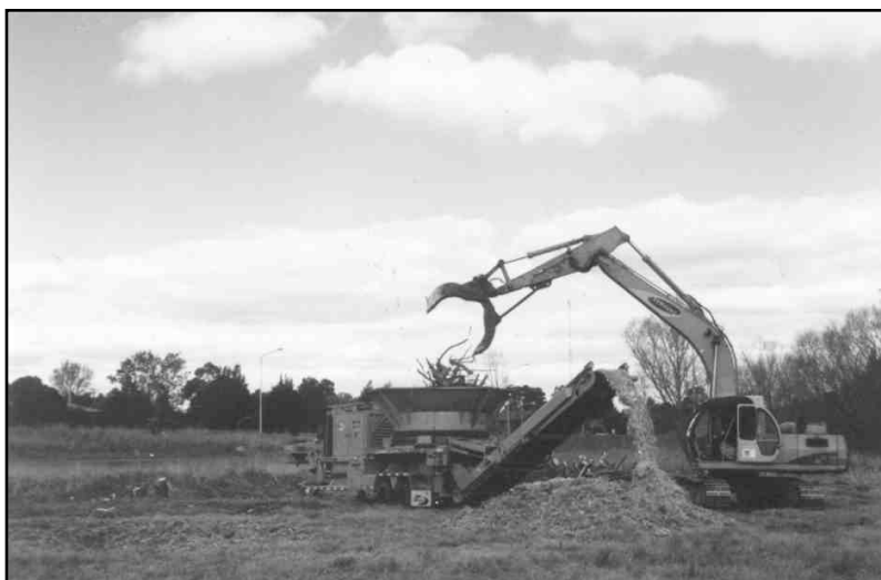
Willow removal and chipping.
