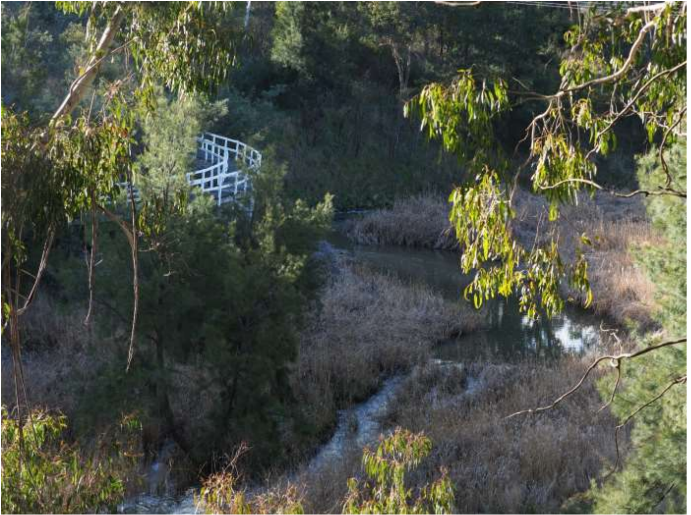
Photo 38: The existing Bridge 1193 from the opposite bank
